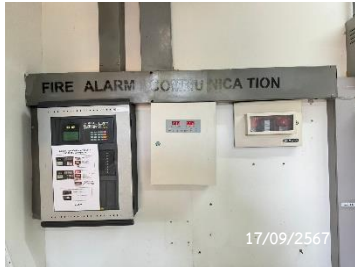
Fire Alarm Control Panel
